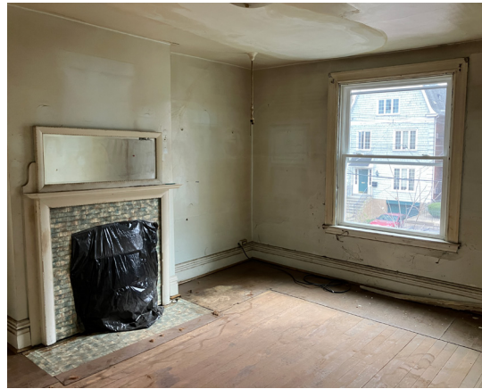
Second Floor: existing southeast bedroom
